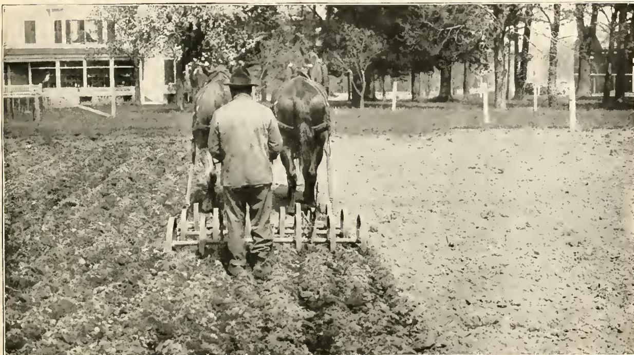
The spring tooth harrow is a good implement for loosening up the soil. Note the efficient work it is doing in this field
