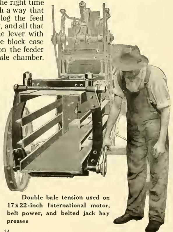
Double bale tension used on 17x22-inch International motor, belt power, and belted jack hay presses
