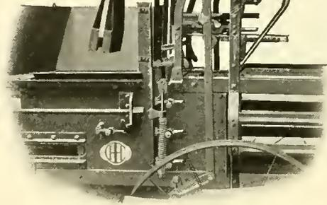
Position after tripping lever. Block case is moved forward
