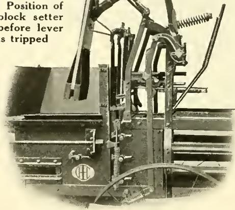
Position after tripping lever. Block case is moved forward
